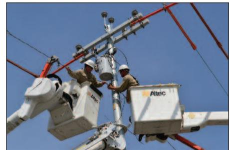
Above, FPU's electric crews work through the spring to upgrade 1.66 miles of three-phase line along city streets and Thornton Taylor Parkway. At top, a crew upgrades a pole in front of FPU's office.
